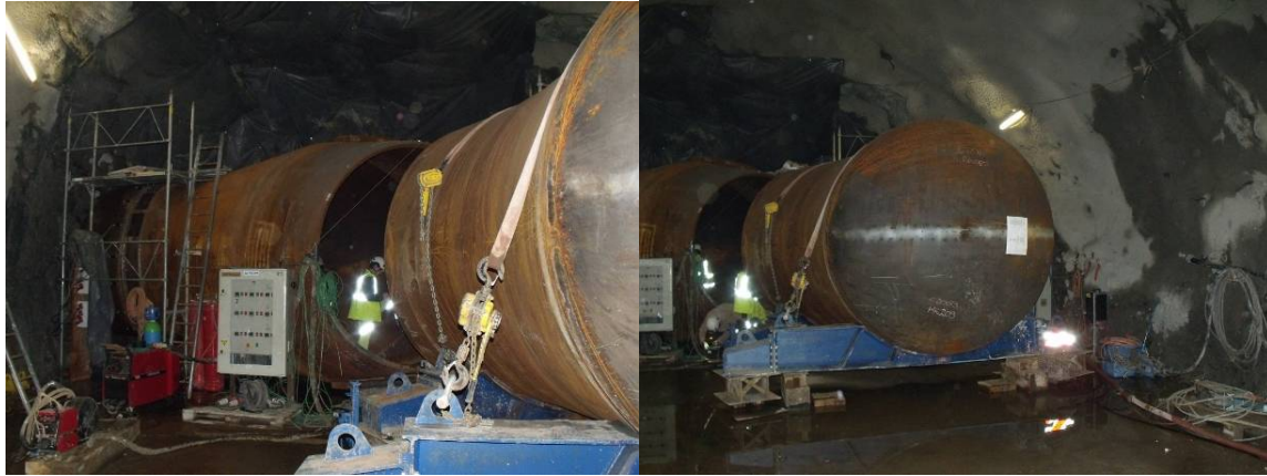
Fig 7. Site pictures of the FMHL+ connecting pipe assembly and welding
